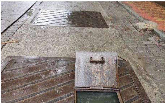
Street view of a flooded valve chamber (undground chambers)
