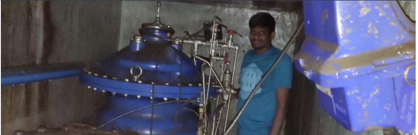
Dorot's local service engineer with a ConDor & 24\"(600mm) valve, after draining the chamber
