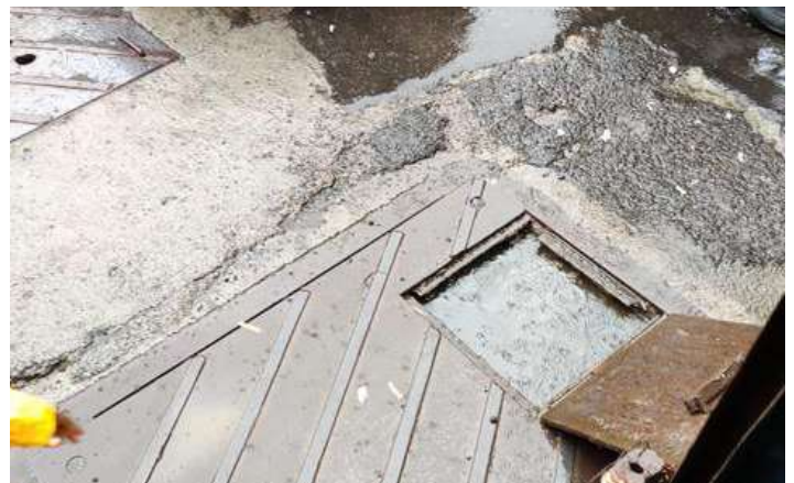
Street view of a flooded valve chamber (undground chambers)
